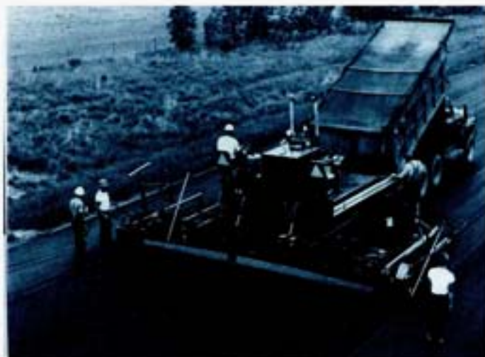
This Matmaker asphalt finisher uses a Screw Conveyor at the back of the tractor unit to move material outward in both directions and spread it uniformly across the entire paving width.
