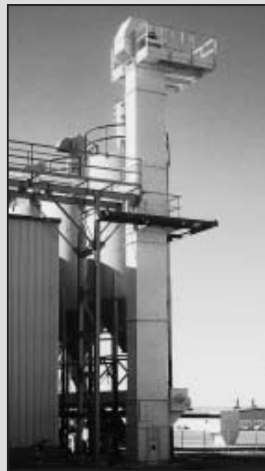
Super Capacity Bucket Elevator at an innovative recycling facility.
